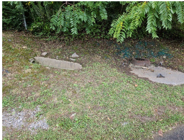
Photo 29: Detention pond retrofit opportunity area
