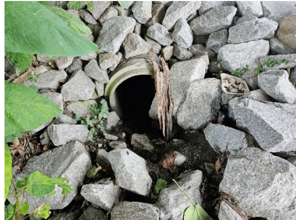
Photo 5: Outfall Chan A
