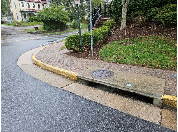
Photo 35: Curb Inlet in Occoquan
