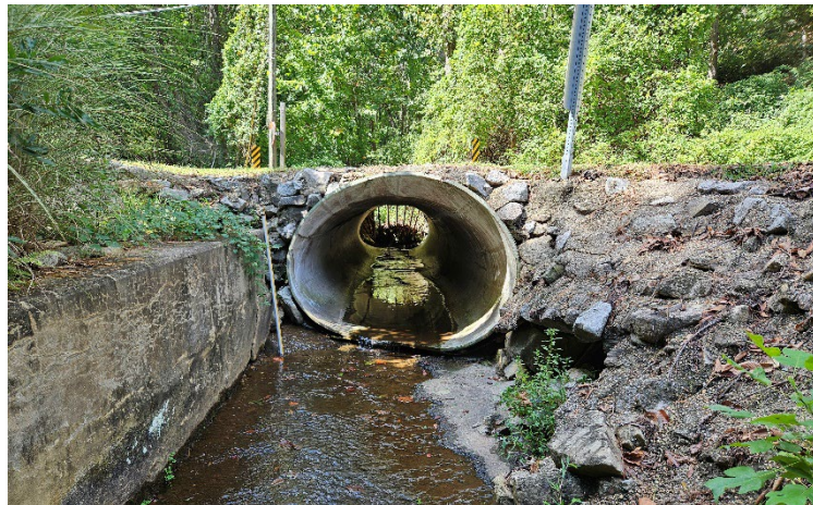
Photo 31: Ballywhack Creek culvert at Union Street
