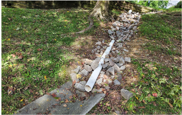
Photo 33: Roof Leader Discharge Pipe and Channel
