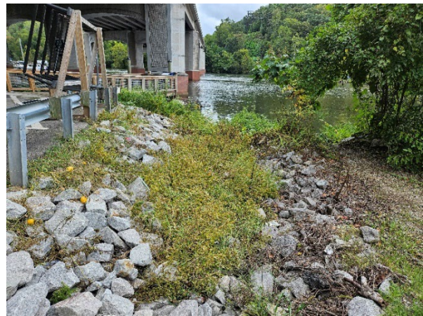
Photo 6: Outfall Chan B
