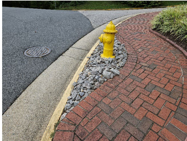
Photo 21: Bioretention opportunity area
