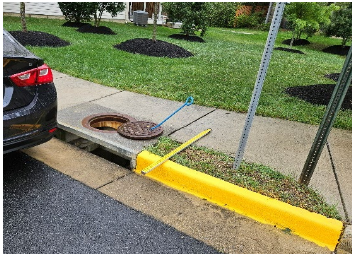
Photo 27: Bioretention opportunity area
