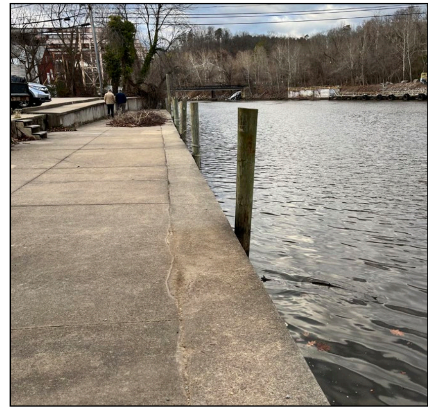
(F) Bulkhead in good condition
