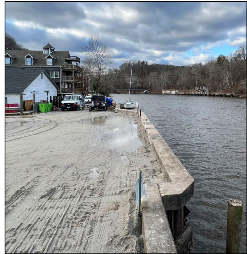
(G) Bulkhead in good condition
