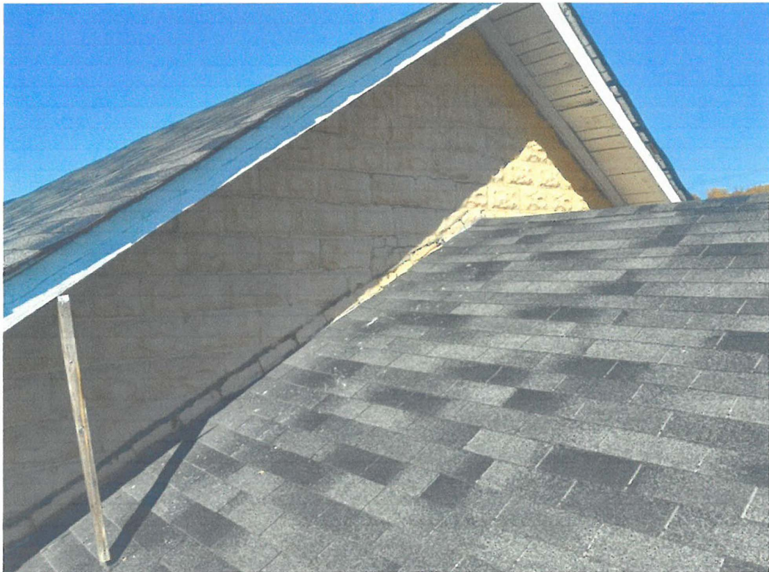
Soffit sealed
